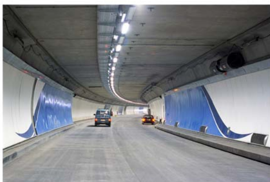
Figure 1.4: Concrete tunnels and road surfaces will stand up to the extreme fire conditions encountered in tunnels.
