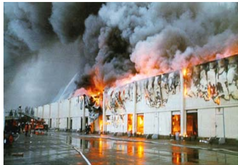
Figure CS8.1: The light-weight sandwich metal panels failed in this abattoir fire in Bordeaux (France) in January 1997. The fire spread throughout the building and to adjacent buildings. (Courtesy SDIS 33, Fire and Rescue Service, Gironde, France)
