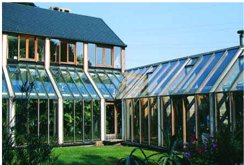
Willem House, Architect Jean Cosse. Using highly glazed south facing façades increases the solar heat gains which this building receives.
