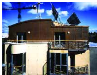
Solar-thermal collectors provide the building with hot water while photo-voltaic panels and wind turbines provide off-grid electricity. Source: Bill Hastings, ARC Digital Photo Graphics
