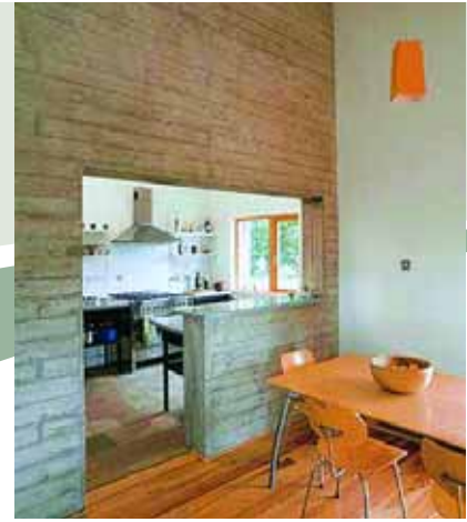
Carton le Vert House, Architect MacGabhann Architects. An internal wall, constructed using high density concrete blocks, is left exposed to provide a high degree of thermal mass.
