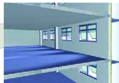
Plain exposed concrete soffits. Plain exposed soffits form part of the thermal mass strategy employed in the James Ussher Library; see case study six. Source: The Concrete Centre
