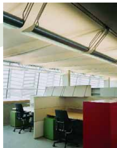
The external façade showing the manually operated ventilator casing and the internal light shelf. The vaulted concrete soffit has been designed to taper up, to maximise the amount of daylight which enters the room. Source: Michael Moran
