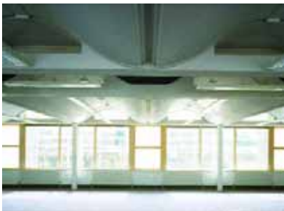
Sinusoidal Slabs used in the BRE building. Source: Fielden Clegg Architects
