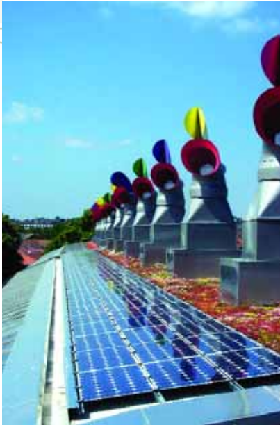
The trademark wind cowls, serve as a crucial element in the developments ventilation strategy. Source: Zedfactory.com
