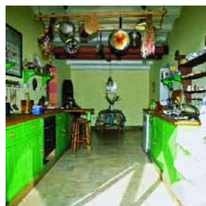
The slab construction is left exposed internally in this room, allowing the walls and ceilings to contribute thermal mass. Additional thermal mass is provided by the tiled floor, which creates a thermal link to the ground floor slab. Copyright: Hockerton Housing Project
