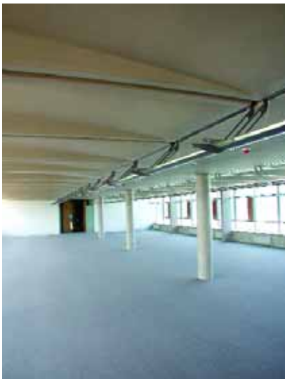
A high quality surface finish is achieved on the slab's undersides and lighting fixtures have been carefully integrated into the ceiling system. Source: Brian Murphy
