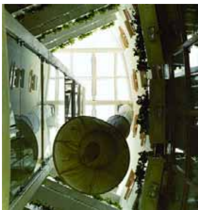
View towards the atrium's skylight, showing the specially commissioned ducting that is used to transport fresh air down to the lower levels of the building. Source: Bill Hastings, ARC Digital Photo Graphics
