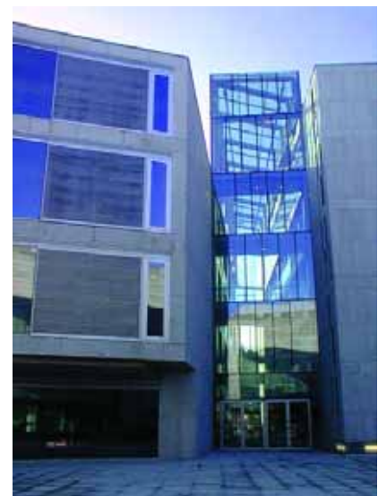
The atrium provides both natural daylight and fresh air to the core of the building. Source: Christian Richters
