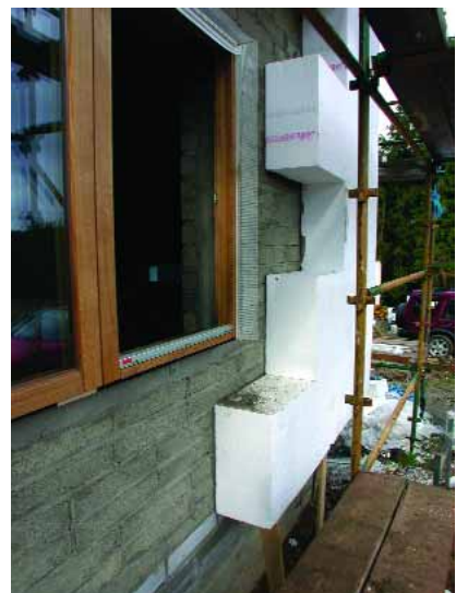
Passive House, Architect MosArt. Externally insulating the blockwork of this building with 325mm of rigid polystyrene ( U -value 0.11 \text{ W m}^2/\text{K} ), not only reduces heat losses, but also improves the effectiveness of the envelope's thermal mass.
