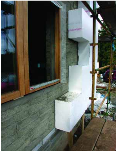
325mm of rigid polystyrene is used to form the external skin of the Passive House. Source: Brian Murphy
