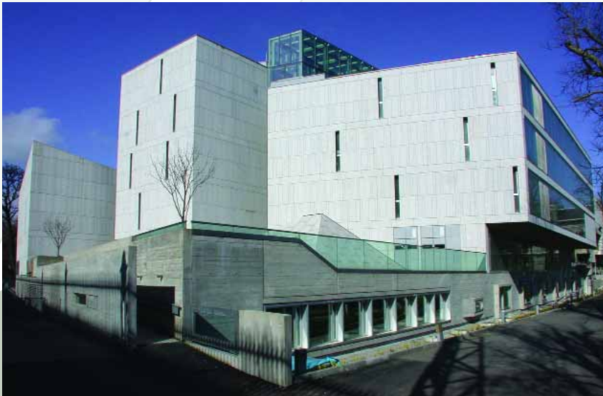
Slit windows have been incorporated into the library's south façade to reduce solar heat gain. Source: Brian Murphy
