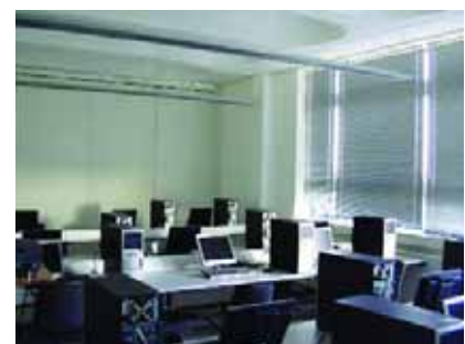
Deeply troughed ceiling soffits provide thermal mass in the buildings computer suites. Source: BDP, Photo: David Barbour
