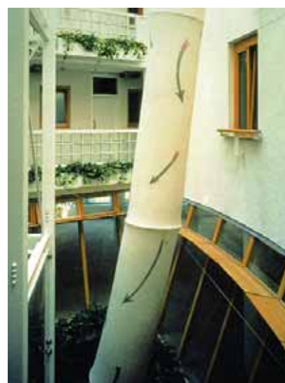
This ventilation shoot was specially commissioned to transport fresh incoming air from the top of the atrium down to the offices on the ground floor. Source: Bill Hastings, ARC Digital Photo Graphics
