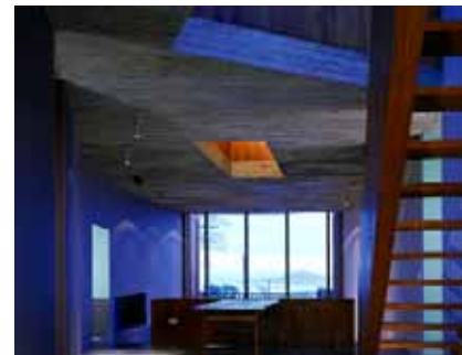
Hawth House, Architect O'Donnell and Thomey Architects. A cast in-situ floor slab provides effective thermal mass in a south facing room. Source: Denis Gilbert/ View Pictures
