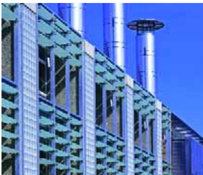
Mechanically actuated louvers, installed on the buildings south facade. Source: Denis Gilbert
