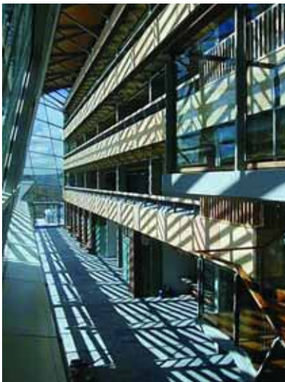
Internal view of the south facing atrium showing the degree to which the external Brise Soleil shades the interior. Source: Michael Moran
