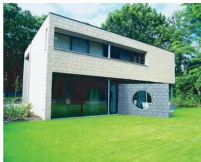
Figure 1d: Concrete block masonry house in Bonheiden, Belgium. (Courtesy Architect – Gie Wollaert, Photographer – FEBE, Belgian Precast Association, Belgium)
