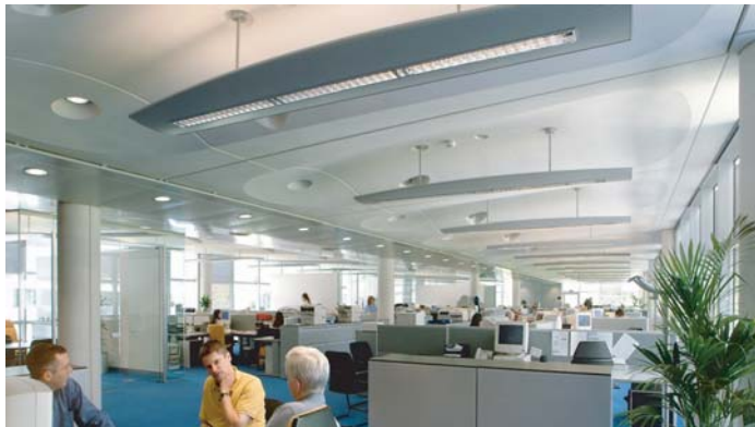
Figure 1b: A comfortable office environment is provided by using concrete's thermal mass to full advantage: Toyota Headquarters, UK. (Courtesy of the Concrete Society, UK)
