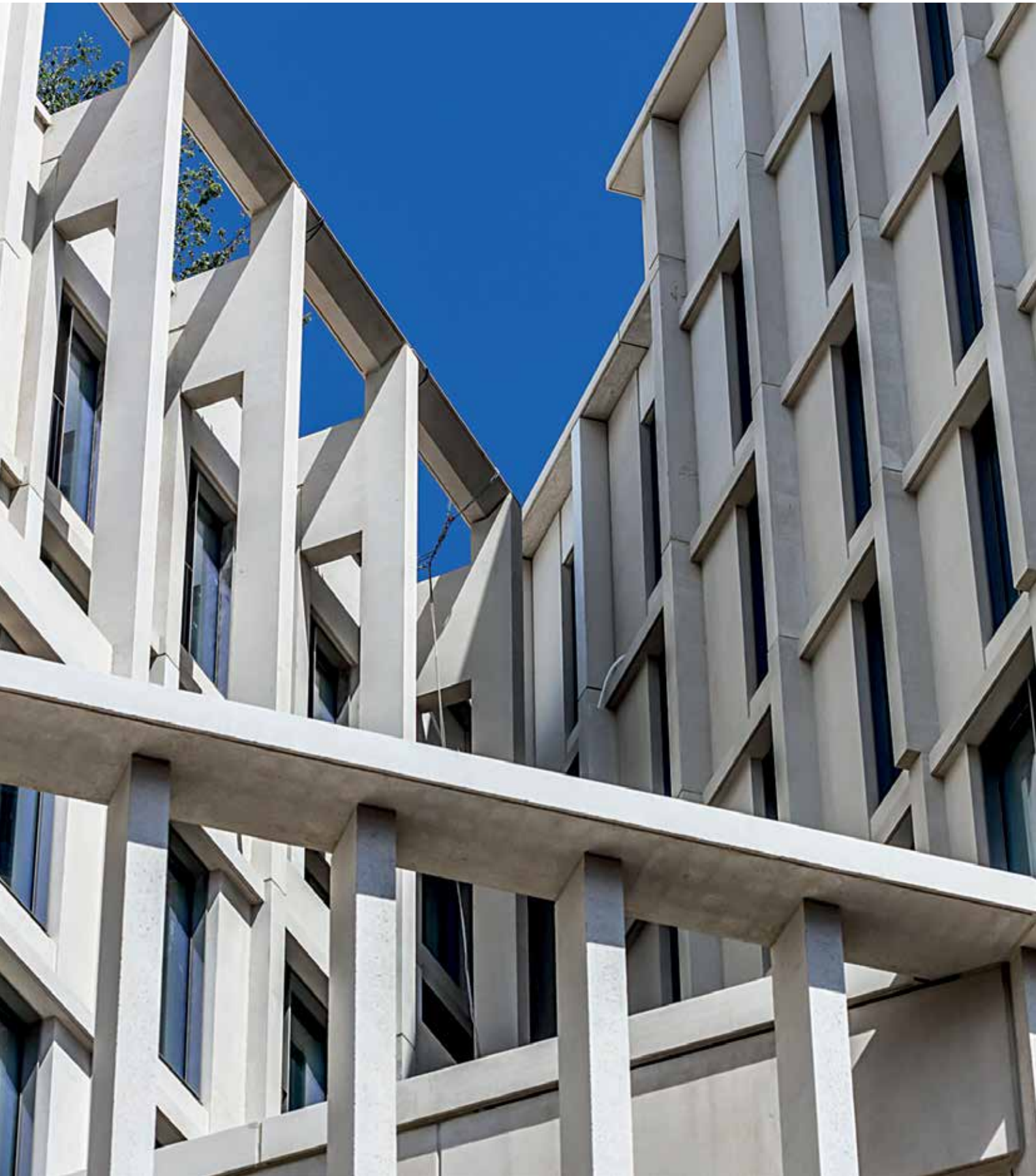
Paul Marshall Building, London School of Economics. Winner International Award, 39th Irish Concrete Society Awards. Irish Precast Concrete Exporter - Techrete.
